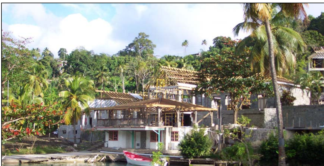
The Central Facilities roof going on
